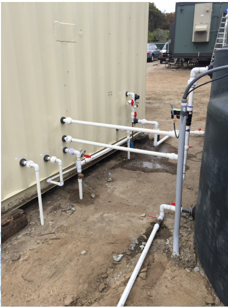
Plumbing and installation by Aqua Clear
